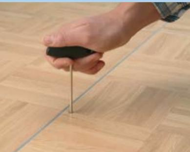
Finally, the appropriate light-metal edging (gold-anodized) is fitted to the outer edges. This is done just as easily as the connection of the individual elements. The bevelled section looks good, is non-slip thanks to its grooved surface, and hence helps to keep your guests safe.
